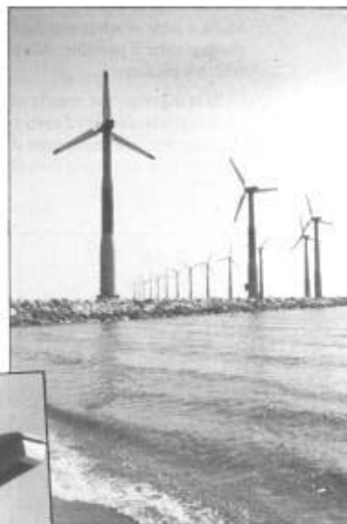
Figure 6 A wind farm in Jutland, Denmark
