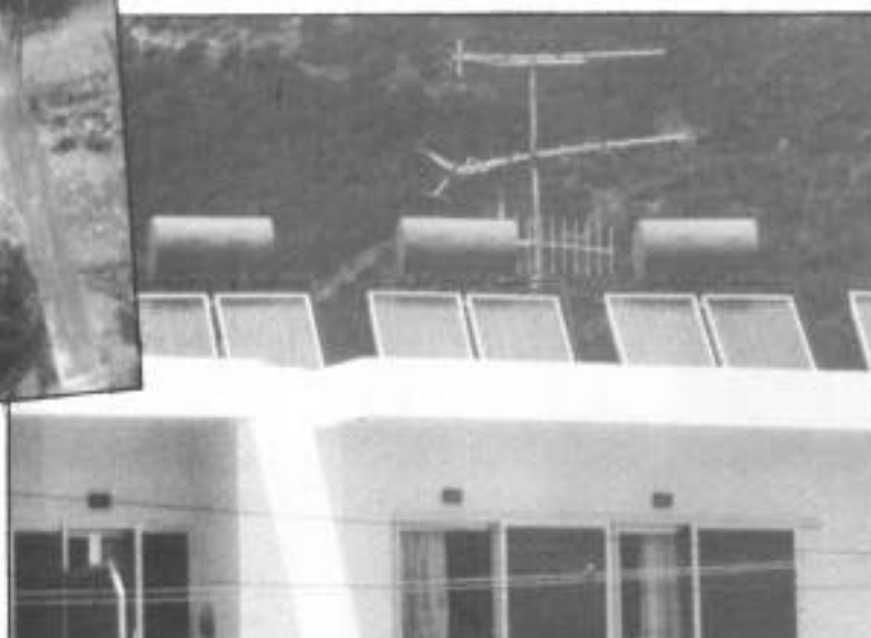
Figure 2 Solar panels using the sun's energy to heat water for a home in Greece
